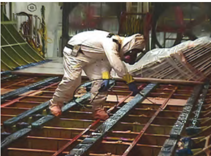
Many operators have repositioned planes to more favorable dry environments. Even so, aircraft can still deteriorate over time in dry storage conditions. Zip-Chem image.
